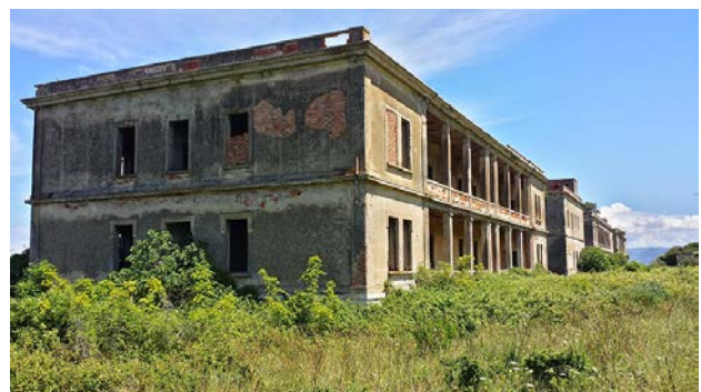
Figure 13. The fronts of the accommodation buildings along the main street
