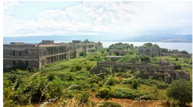
Figure 12. View of the complex
