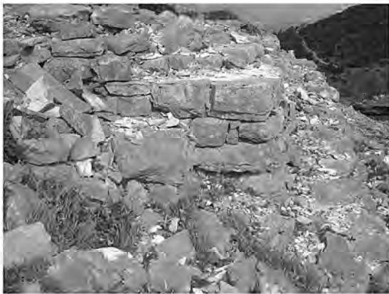
Figure 2: Tower of the fortified Settlement of Paleospiti.
