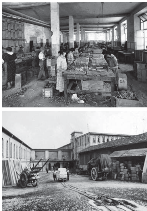
Figs. 3a-b. Interiors of the establishment and storehouse, late 19 th century (Pigna Paper Mill Historical Archive).
