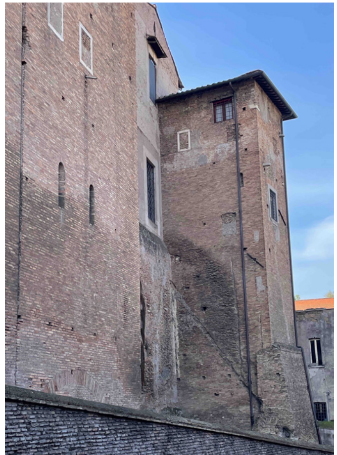
Figure 6. Rome, Santi Quattro Coronati, cardinal residence, the presumed latrine tower on the right (Autor).
